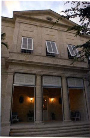
nearly-completed entry portico at evening
