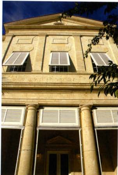
nearly-completed entry portico by morning
