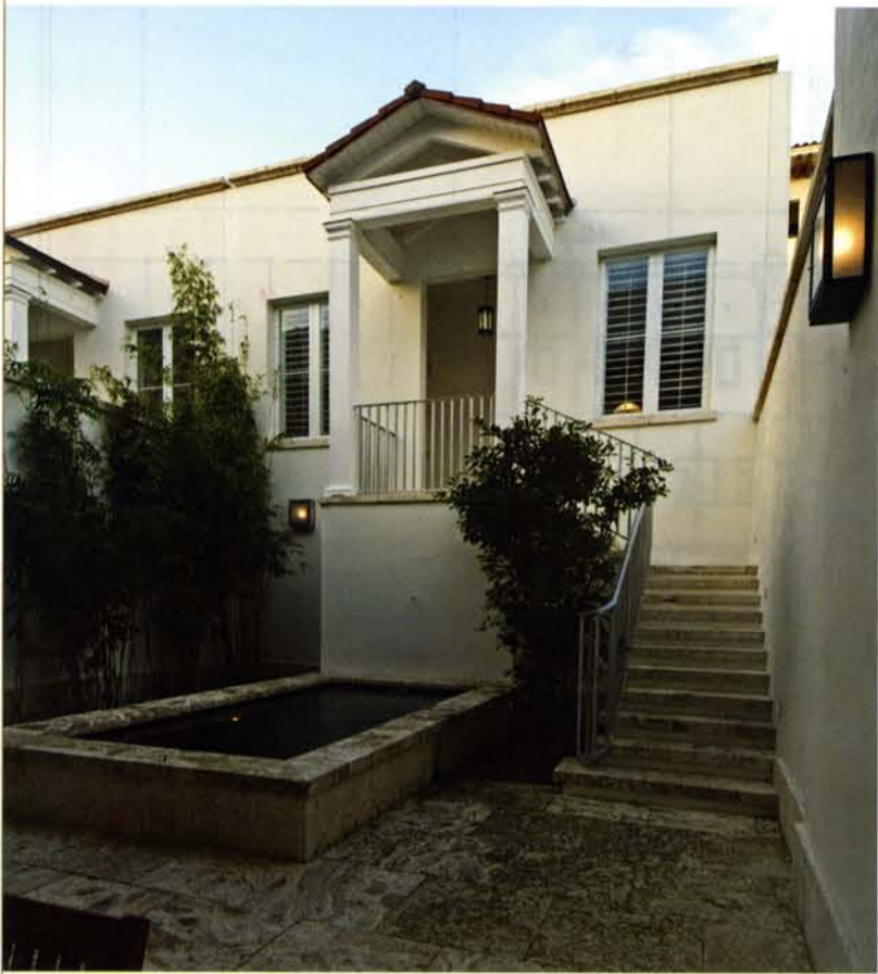
Above and right: The central courtyards, which separate the main houses from the rear garage structures, include small pools and provide the houses with light and ventilation.
